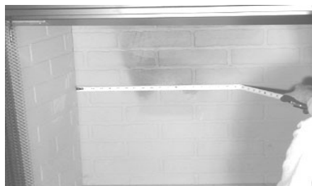
Figure 1 Measure Firebox
